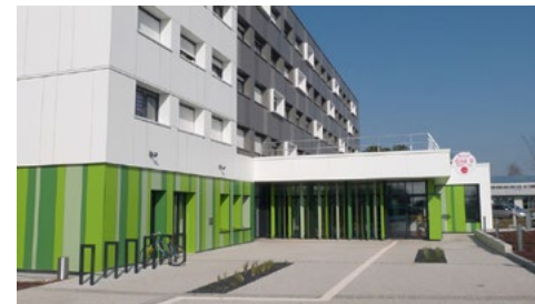
Front desk of the campus 1 residence
